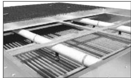
Drift Eliminators Removed for Coil Inspection
